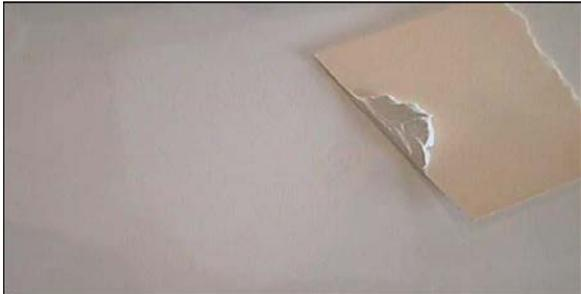
Begin by wiping the area clean with acetone. Mix 10-12 drops of catalyst with 1 ounce (half a jar) of Spectrum Color factory color matched Patch Paste®. Fill the damaged area with the smooth drag. A second application may be necessary. After patch paste is cured, 1-2 hours sand and buff to finish.
